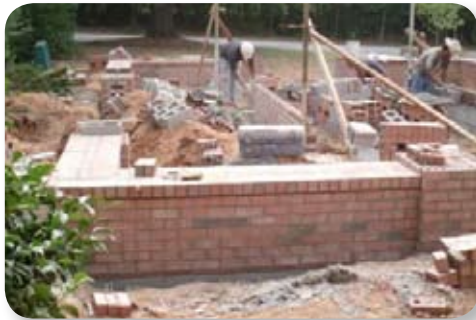
Alliance Meditation Garden under construction earlier this summer
